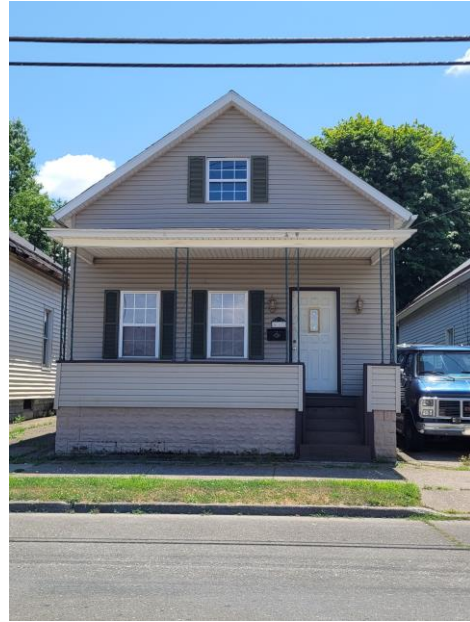
518 West 19th Street (before rehab)
